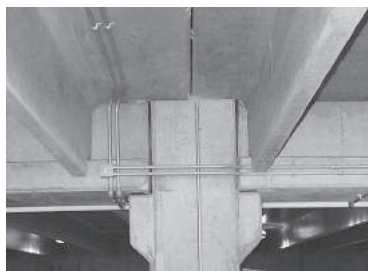
Concrete smooth or "roller" support.
