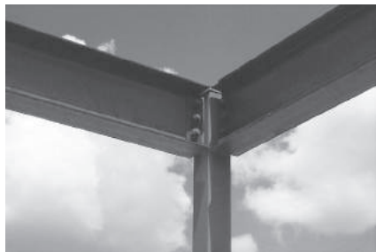
Pin-connected steel members.
